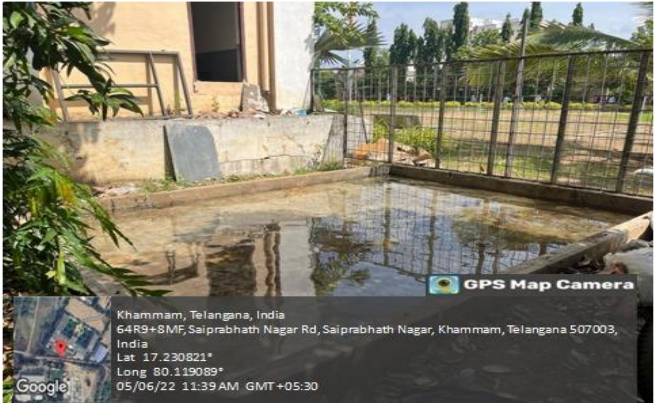
Fig 12: Bund for Rain water storage
