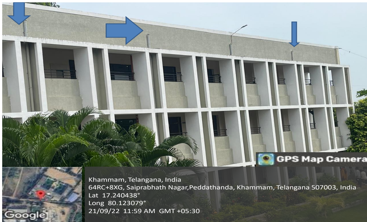
Fig 3: Rainwater collecting through pipelines for harvesting
