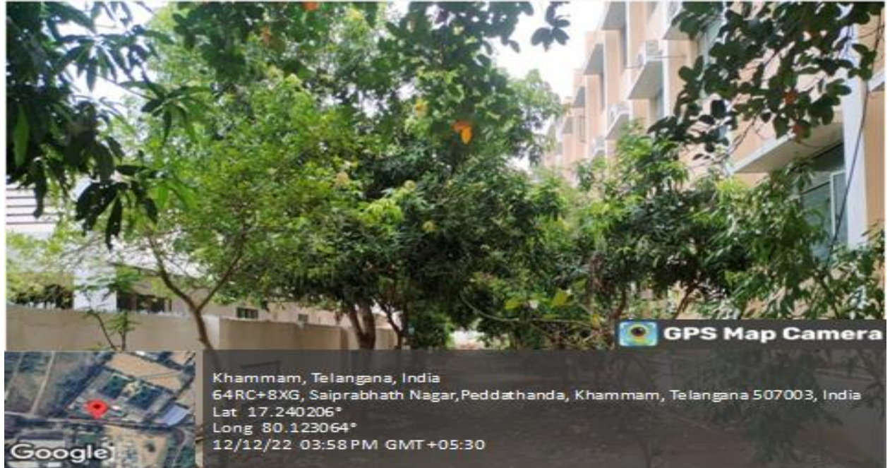
Fig 5: Rainwater collecting through pipelines for harvesting
