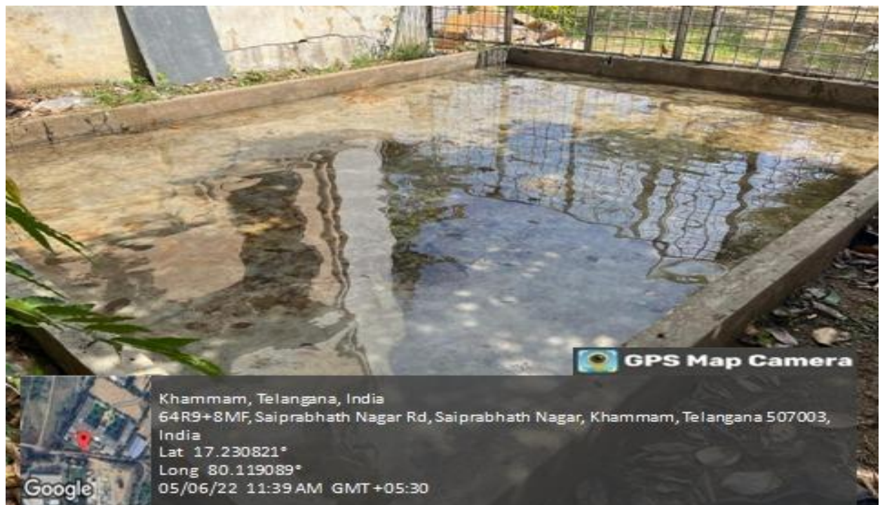
Fig 11: Bund for Rain water storage
