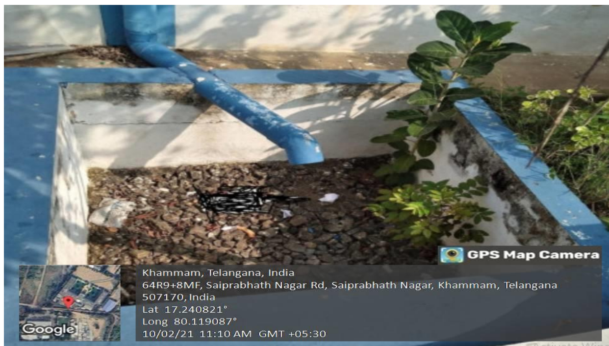
Fig 2: Rain Water Harvesting Pit
